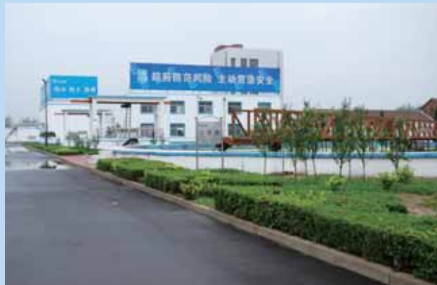
Ling County Waste Water Treatment Project 陵縣污水處理項目
