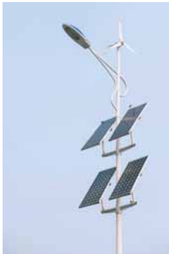
Wind-solar hybrid streetlights 風光互補的節能路燈
