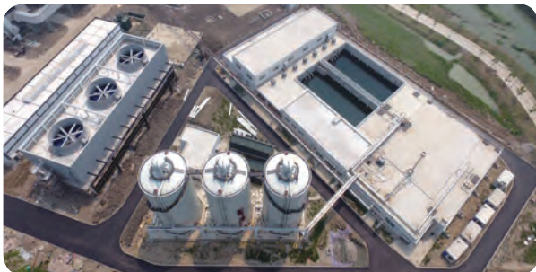
Leachate treatment system 成套滲濾液處理系統
