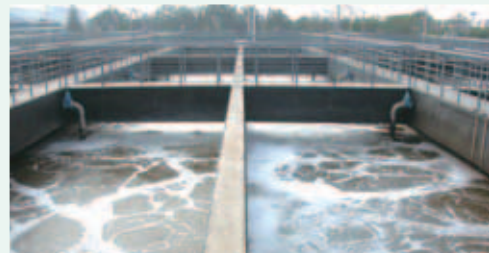
Jiangyin Chengxi Waste Water Treatment Plant 江陰澄西污水處理廠
