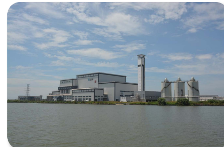
Wujiang Waste-to-energy Project
