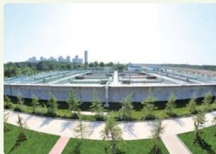
Ji'nan Waste Water Treatment Project
