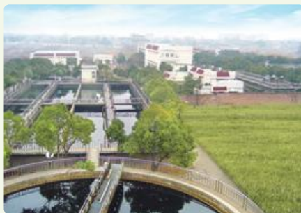
Jiangyin Waste Water Treatment Project
