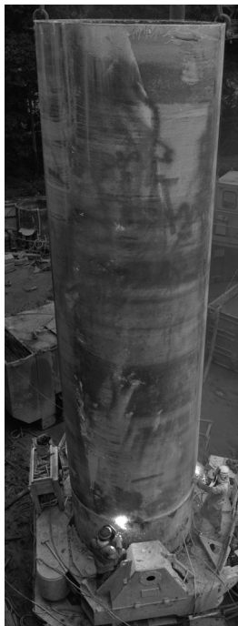
Temporary steel casing to be driven into the ground
