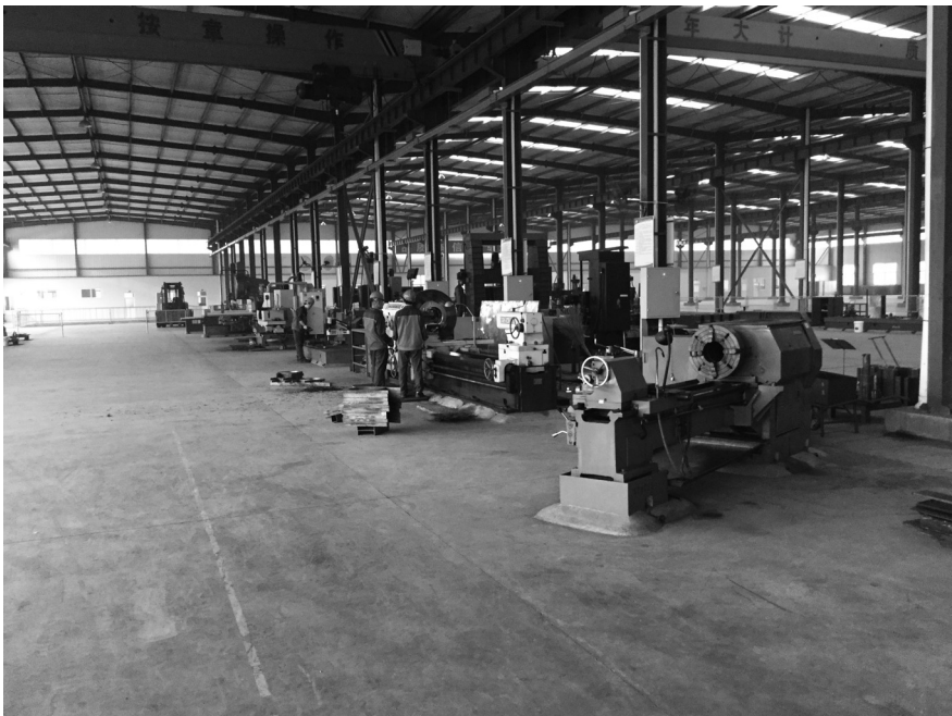
Production Base of Shandong Dereton
