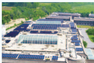
Rooftop photovoltaic panels
