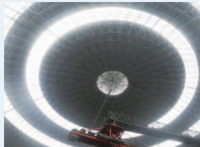
Photo "Round-shaped of Coal Yard", by Ye Junjie from Shangqiu Power Plant
