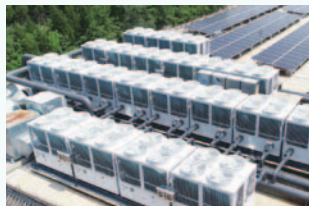
Low-temperature air source heat pump
