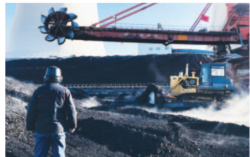
Fuel supply was ensured
