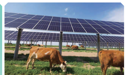
Husbandry and Photovoltaic Complementary Photovoltaic Power Generation Project
