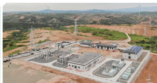
CP Chaoyang 250MW Integrated Intelligent Wind-and-Energy Storage Power Generation Project
