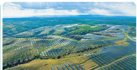
Xinrong Phase II 600MW Grid Parity Photovoltaic Power Generation Project
