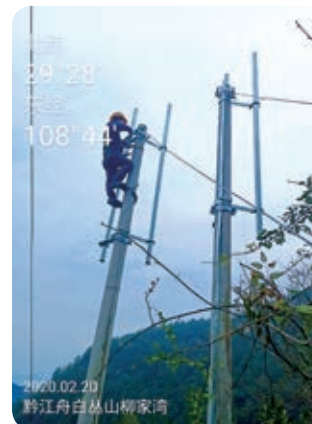
▲ Construction workers are constructing base stations in mountainous areas
