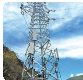
▲ Using power tower to mount mobile network antennas
