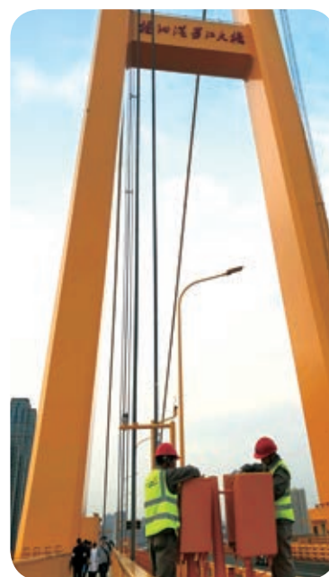
▲ Construction site of river-spanning bridges
