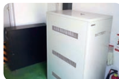
▲ Placing equipment for backup power supply, monitoring and power generation equipment
