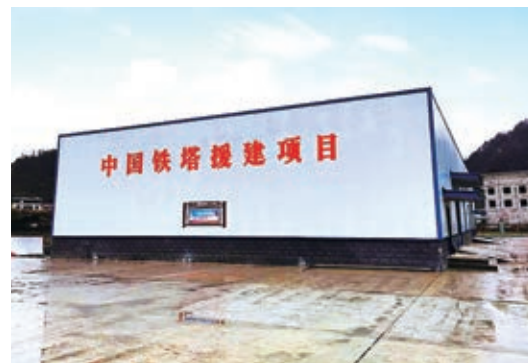
▲ China Tower-aided tea factory
