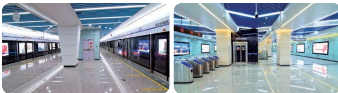
▲ 5G network DAS coverage in Chengdu Metro Line 10
