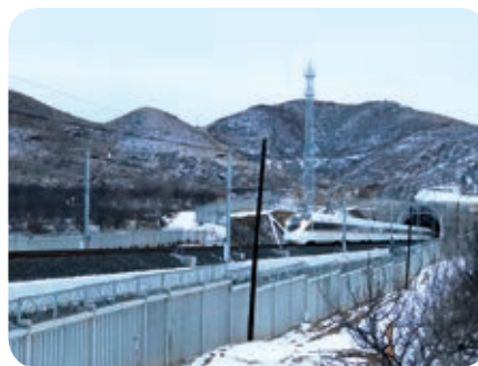
▲ Using railway telecommunication tower for signal coverage
