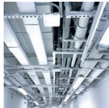
▲ DAS construction in an Olympic venue
