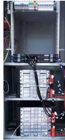
▲ Scenario of cascade utilization of power batteries for base stations
