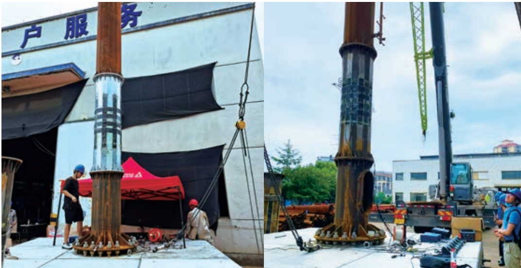
▲ Reinforcement of existing tower sites with carbon fiber
