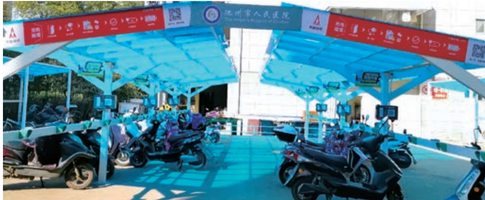
▲ Community battery charging piles
