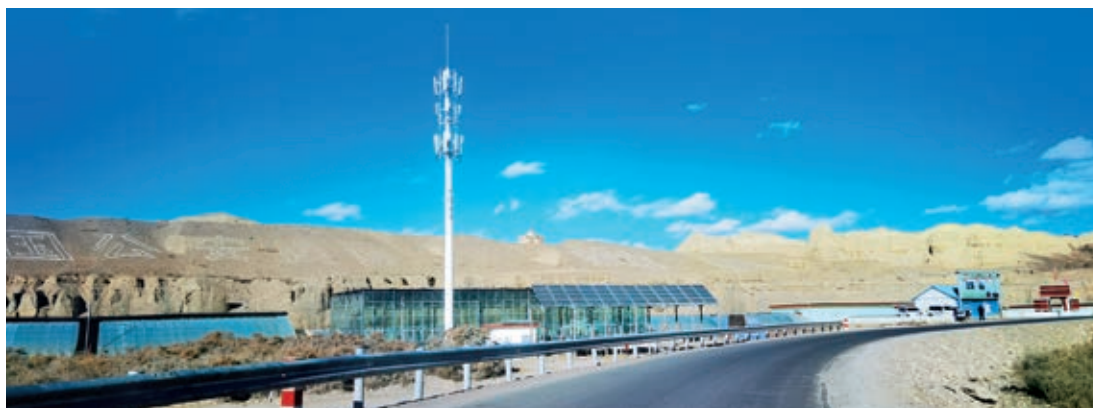
▲ A wind-solar hybrid power base station in Naqu
