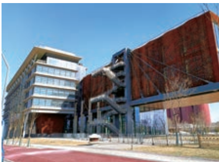
▲ Business complex in Shougang Park, Beijing
