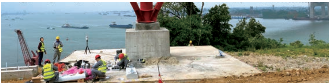
▲ Mounting telecommunications antennas on the river-crossing 220 kV power tower
