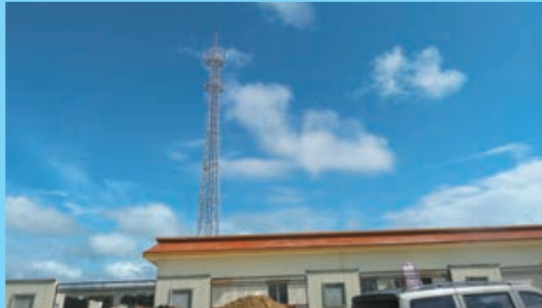
Deploying antennas on shared railway network towers
