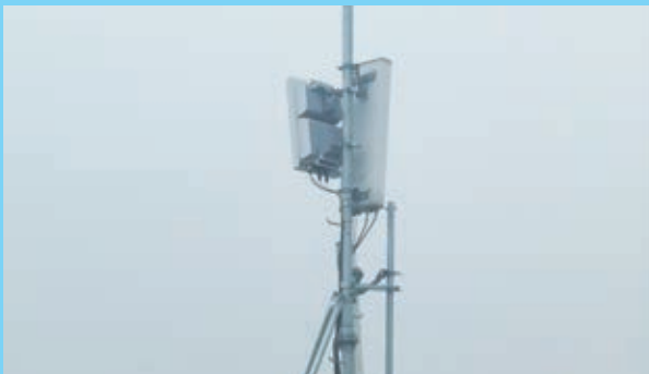
Deployment of 5G facilities on the rooftop of Sichuan Provincial Government
