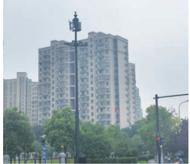
Replacement of mid pole lights
