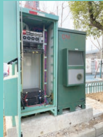
Recycle site of dismantling the old switching power supply
