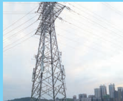
Sharing power tower to solve difficulty in location selection of relocation areas
