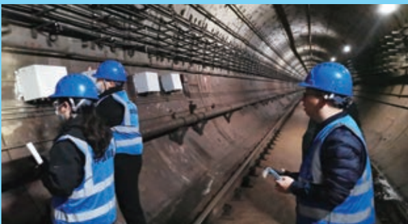
Construction of Nanjing Metro Network
