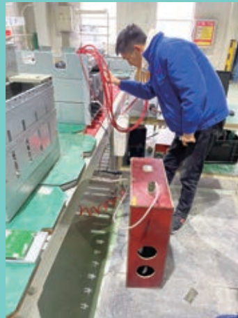
Transformation test of dismantling the old switching power supply
