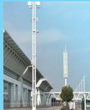
Construction of telecommunication towers using light poles
