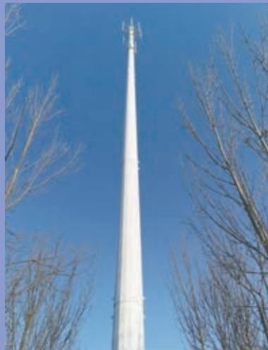
Example of low-cost single tube tower application
