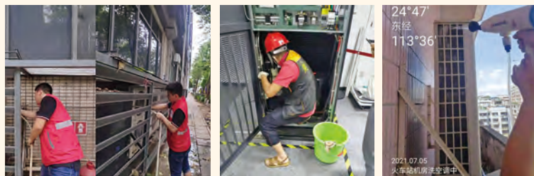
Carrying out green and low-carbon equipment room reconfiguration
