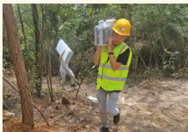
Base station construction in Wulong poor remote mountainous area
