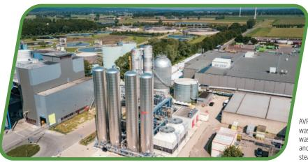
AVR treats waste including biomass, industrial wastewater, municipal solid waste, commercial waste, and hazardous waste, all of which are treated and converted into energy – namely electricity, steam and heat.
