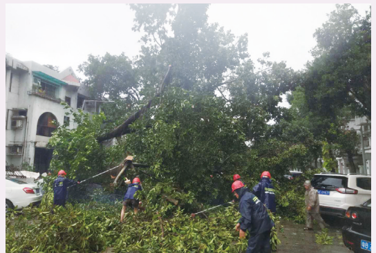
Panyu property management staff engaged in emergency repair and restoration
