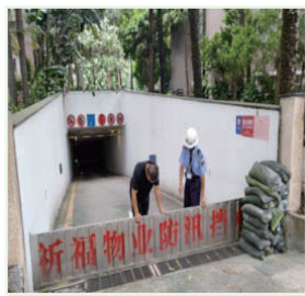
Placing flood barriers and sandbags
