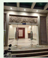
Downlight renovation (after)
