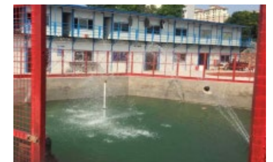
Rainwater collection facility in the living area in the construction site
