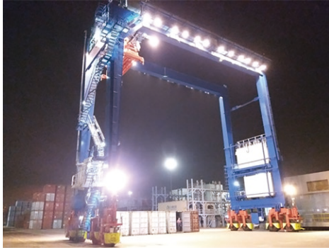
Curtain Wall Lighting System Project in Jinzhou New Age Terminal.
