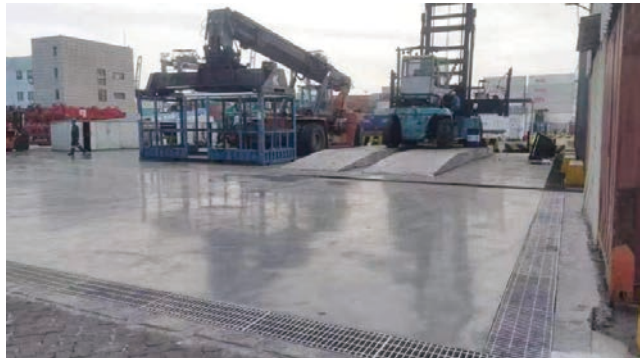
The sewage recycling facility in Xiamen Ocean Gate Terminal is used to collect, precipitate, and reuse the sewage after vehicle cleaning.
