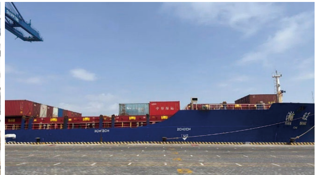
Quan Zhou Pacific Terminal has deepened cooperation with logistics companies to improve its terminal container services.
