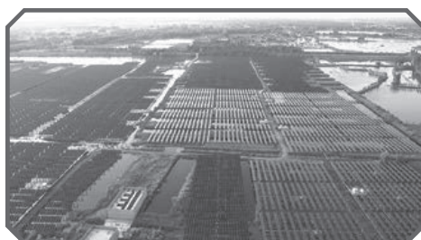
Centralised Photovoltaic Power Plant, Weishan County, Shandong Province
