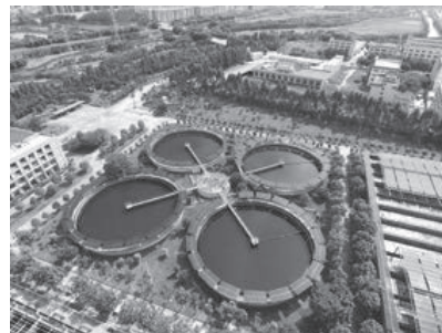
Distributed Photovoltaic Power Plant in a water plant of BEWG, Dongguan, Guangdong Province
