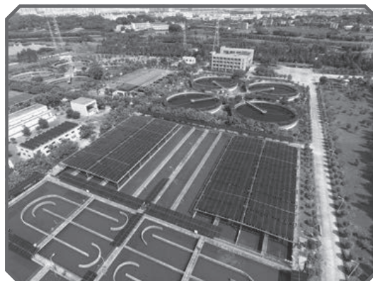
Distributed Photovoltaic Power Station in a water plant of BEWG, Dongguan, Guangdong Province
