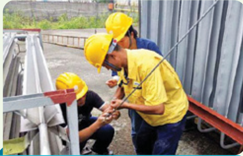
ENN Taizhou employees repairing damaged equipment
