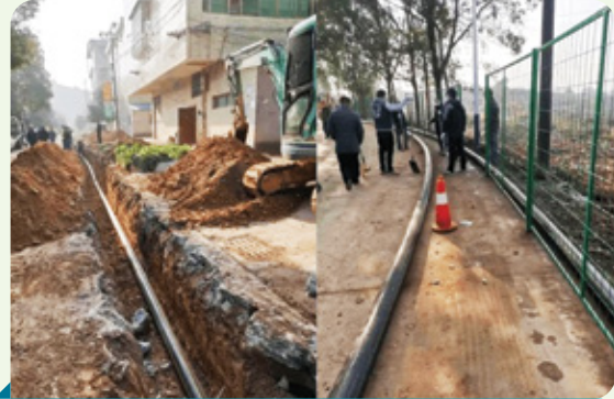
ENN Changsha laying a pipeline for the hospital
