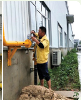
Maintaining pressure-regulating equipment
