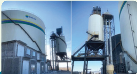
Daqing Ubiquitous Energy Station reduces fly ash pollution
