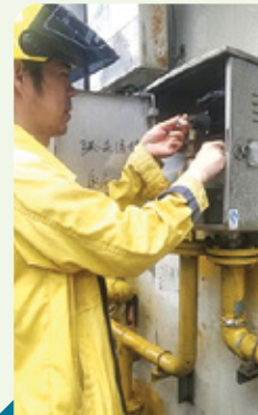
Maintaining pressure-regulating equipment
