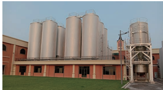
Turnkey project of beer brewing
