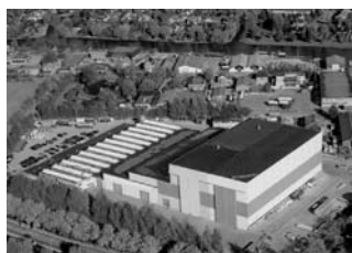
Holvrieka Group factory premises in Sneek, the Netherlands
