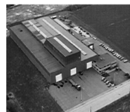
Holvrieka Group factory premises in Menen, Belgium
