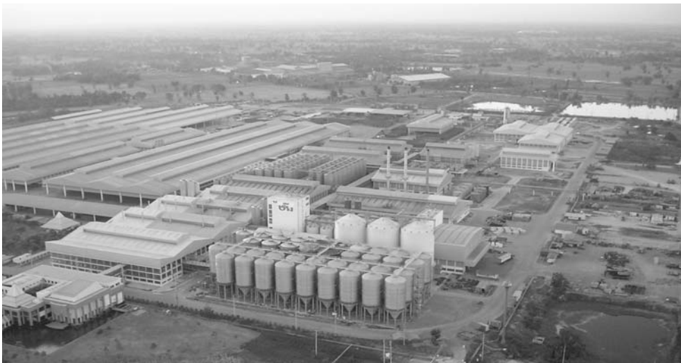
Beer processing and distribution turnkey project Manufacturer and constructor: the Holvrieka Group
