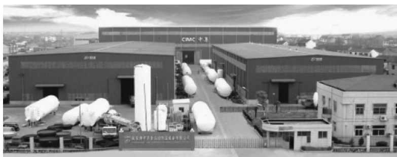
Zhangjiagang CIMC factory premises at Xiangshan Road, Zhangjiagang
