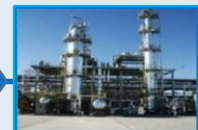
液化工厂 H2 liquefaction plant
