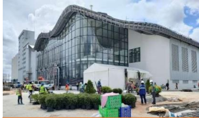
Turnkey brewery and experience center, Cambodia
