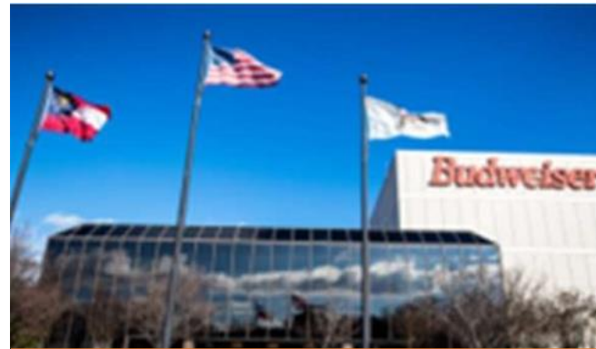
Process design & equipment for brownfield & hard seltzer facility, USA
