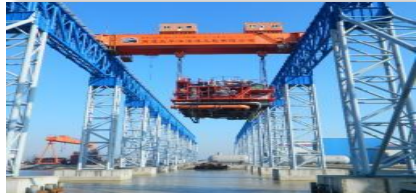
▲ Offshore oil and gas processing module
