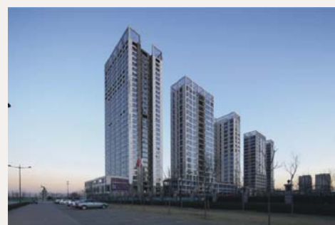
Tianjin Hailrun Plaza
