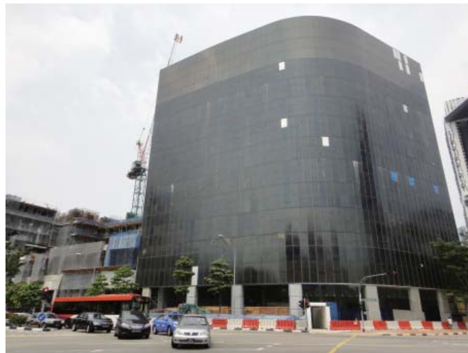
View from intersection of New Bridge Road/Outram Road/Cantonment Road
