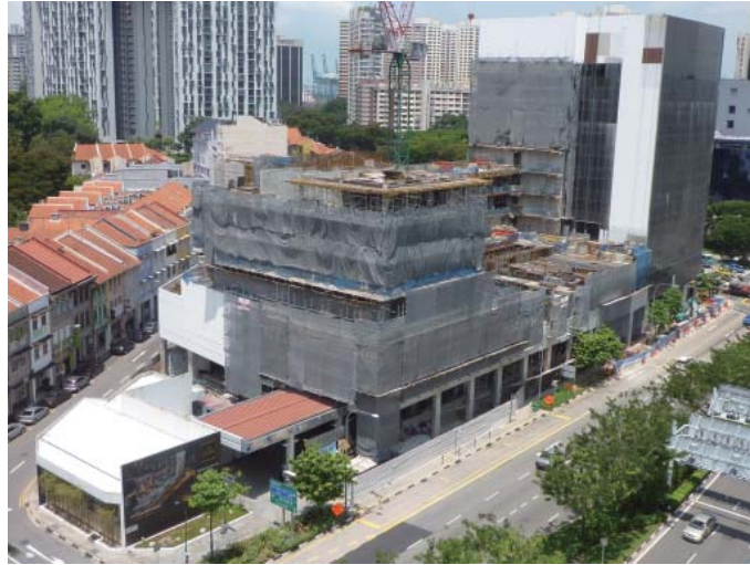
Aerial view of whole development
