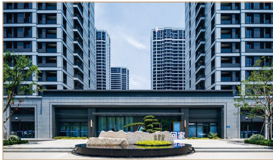
杭州沁香公寓 Hangzhou Qinxiang Apartment
