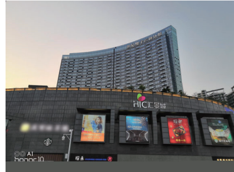
The outlook of Huijing City is featured with large advertising signboards with lighting effects at night and the entrance is also decorated with curtain walls.
