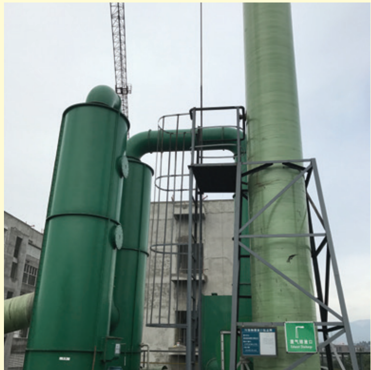
重慶康樂製藥有限公司處理廢棄物設施 — 車間廢氣治理設施 Waste disposal facility of Chongqing Kangle Pharmaceutical Ltd. — Waste gas treatment facility
