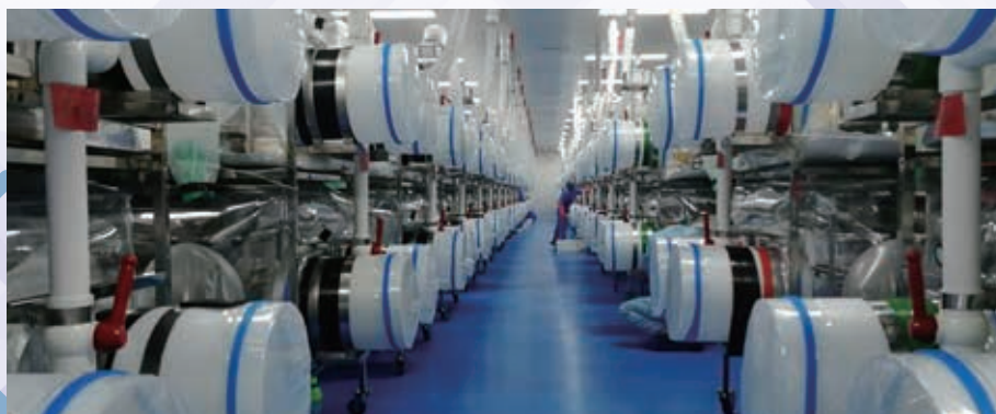
斯貝福之生產車間 Production plant of SPF
