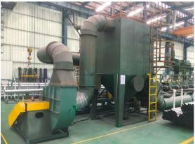
Guangzhou Mayer's production plants are equipped with dust collectors with pulse jet filter bags, which adopt automatic dust cleaning devices to maintain the stable filtering effect of the dust collectors and thus to reduce particles and dust emissions during production.
