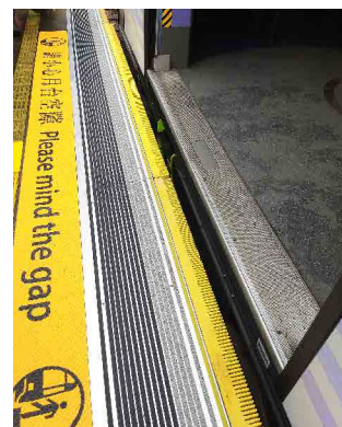
Board Easy Mat installed for trial at Goodview Garden Stop
