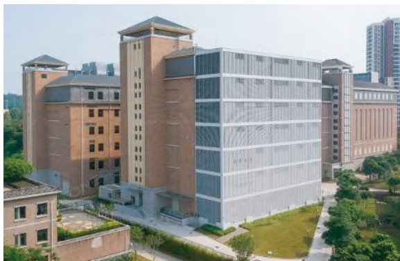
Ping An Guanlan No.3 Data Center
