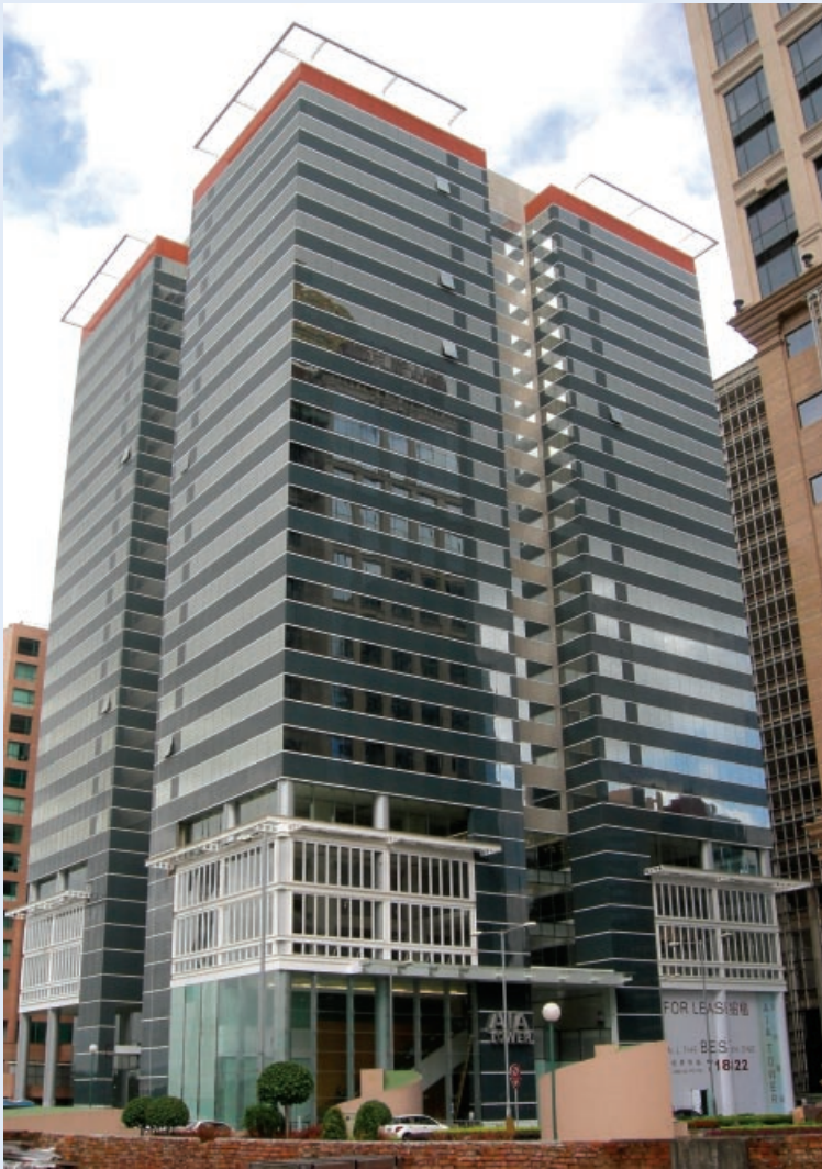
AIA Tower, Macau
