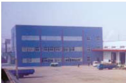
The warehouse in the Jiuting Industrial district, Shanghai has a gross floor area of 17,474 sq.m.
