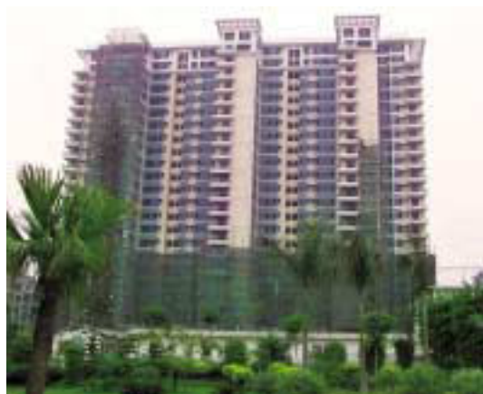
Phase 1, Westmin Plaza in Guangzhou, a commercial/residential development totalling around 40,000 sq.m.
