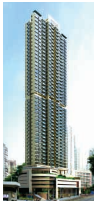
Po Kong Village Road project
