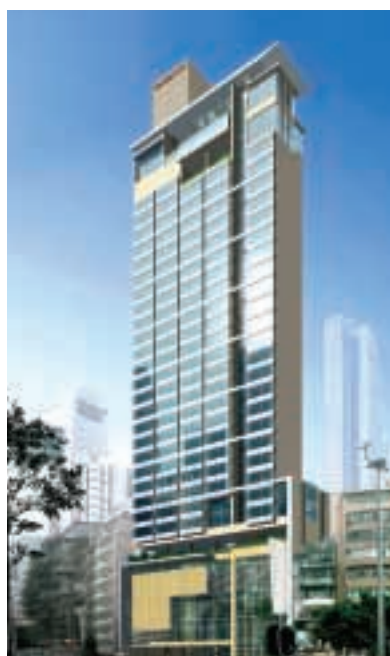
Leighton Road project
