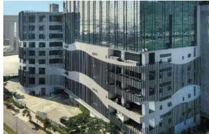
Vehicular ramp access to every warehouse floor
