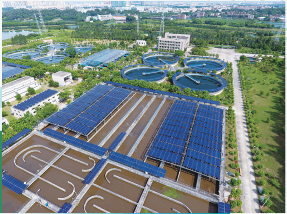
Distributed photovoltaic power station in a water plant of BEWG, Dongguan, Guangdong Province 廣東省東莞北控水務集團水廠內的分佈式光伏發電站
