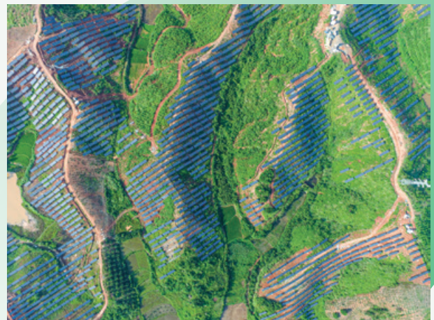
Centralised photovoltaic power plant, Jinzhai County, Anhui Province 安徽省金寨縣集中式光伏發電站
