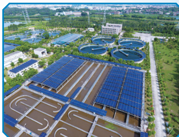
Distributed Photovoltaic Power Station in a water plant of BEWG, Dongguan, Guangdong Province
