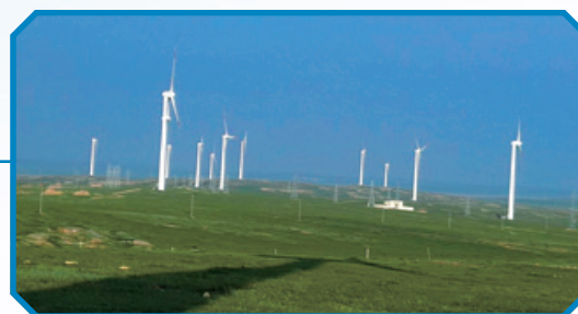
Wind Power Plant, Baotou City, The Inner Mongolia Autonomous Region
