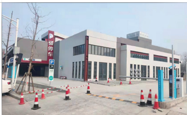
Nanjing Lianhua Village Parking Garage Project* 南京蓮花村立體停車庫項目
