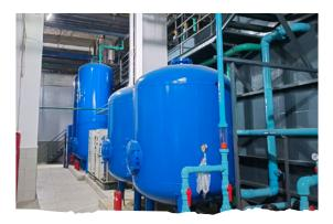
INDIGO's existing grey water system collects high-quality wastewater and rainwater to make grey water for toilet flushing and greenery irrigation. Cutting-edge treatment technology can effectively treat sewage water, allowing it to reach grey water or even pure water standards for use in cooling towers. In 2022, INDIGO built a sewage water recycling system, further improving our water savings and reducing wastewater discharged into the municipal pipework system.
