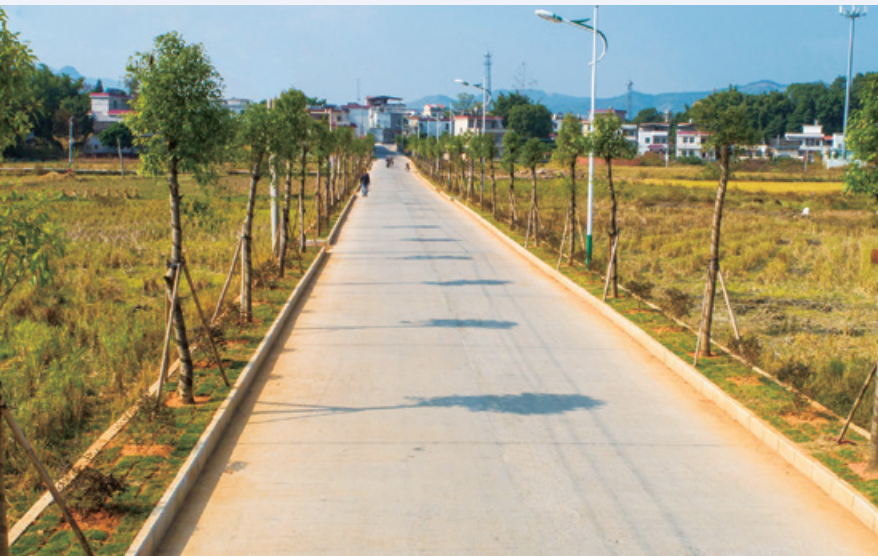
Newly-built village roads and solar street lights
