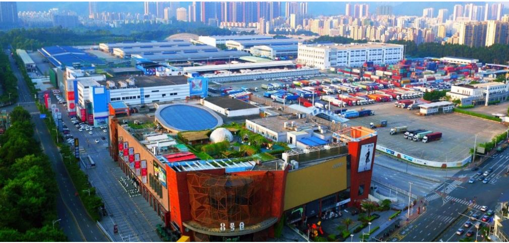
Photo of South China Logistics Park
