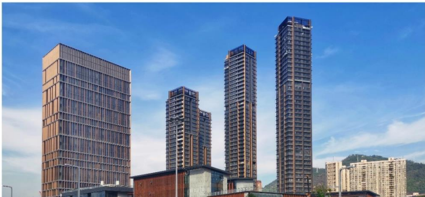
Real image of the first phase of the Qianhai Project
