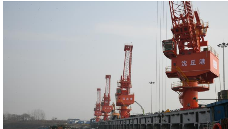
SZI Port (Henan Shenqiu) (real image) The first vessel successfully berthed and underwent heavy load testing at the end of 2022.
