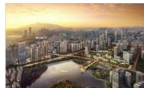
SZI-South China Logistics Park Project
