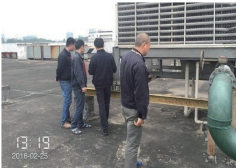
Special safety examination of power equipment
