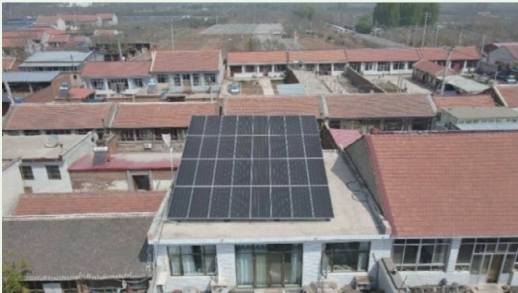
▲ An 18KW Distributed Photovoltaic Project in Zaozhuang, Shandong Province
