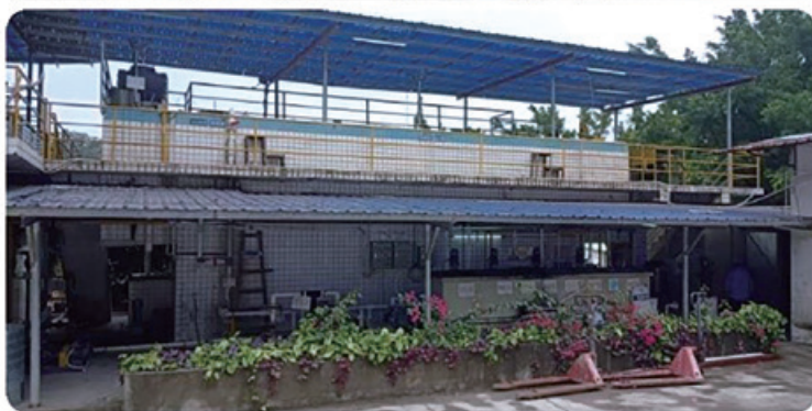
Electroplating wastewater treatment station and other sewage treatment stations in the plant area
