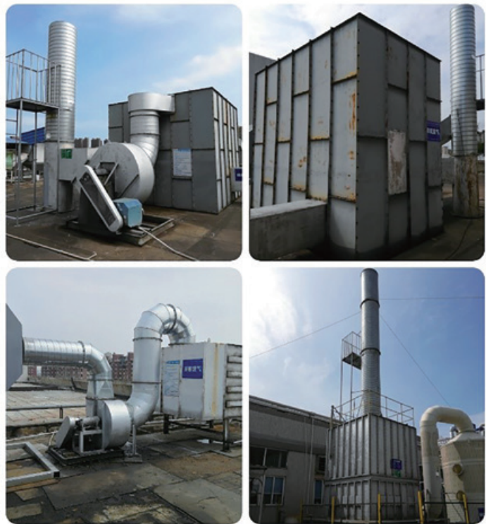
Activated carbon absorption devices at each discharge outlet within production plants 廠房內各廢氣排放口的活性炭吸附裝置
