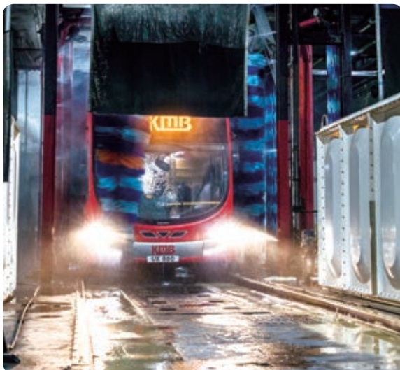
Our depots are equipped with automatic waste water treatment systems
