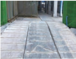
Surface protection of sealing construction road
