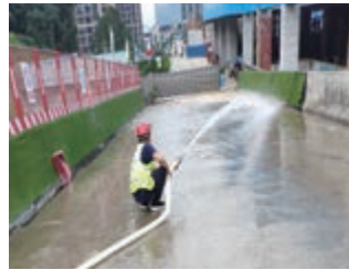
Construction road flushing
