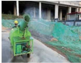
Spraying with fog gun and covering with bare soil
