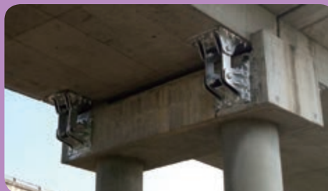
▲ Addition of Anti-draw-out Piles
